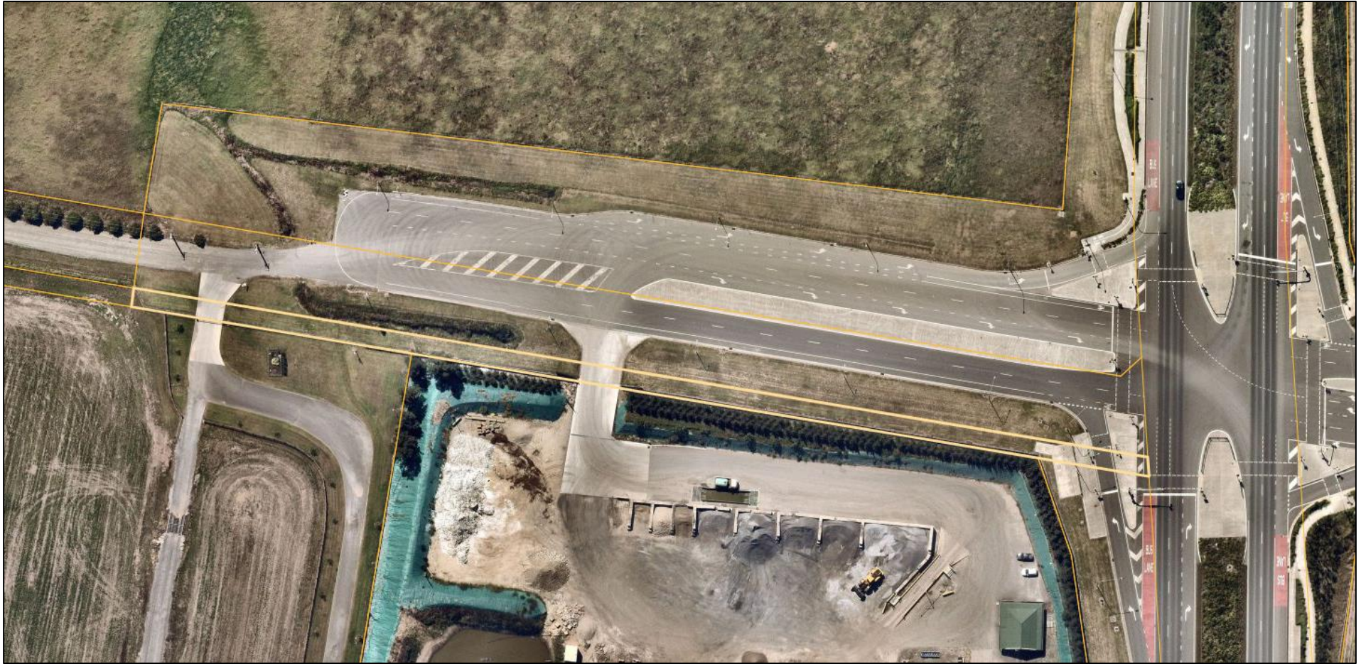
Figure 15: Maryland's Link Road 2.
